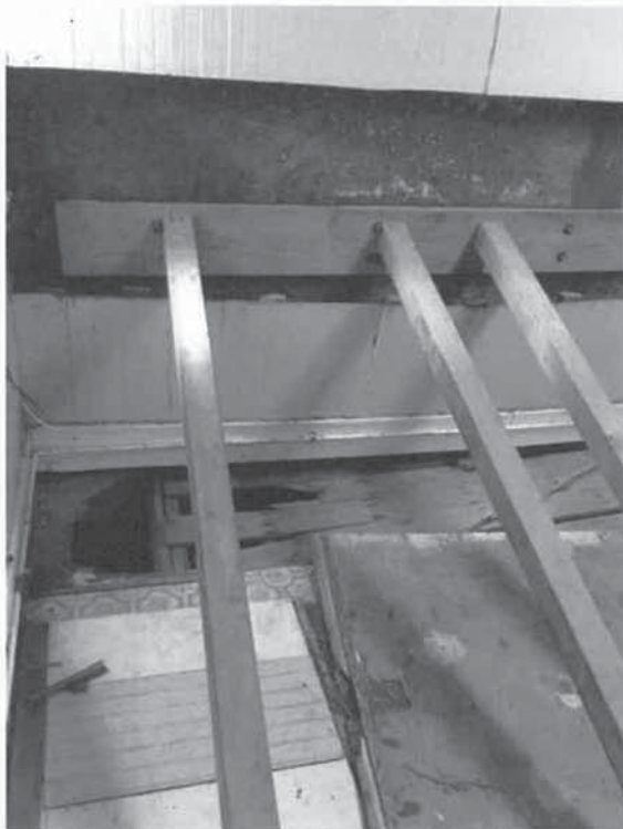
Photo 5 & 6: Close up of the failed retaining wall and insufficient waterproofing which led to the dry rotting floor framing.
