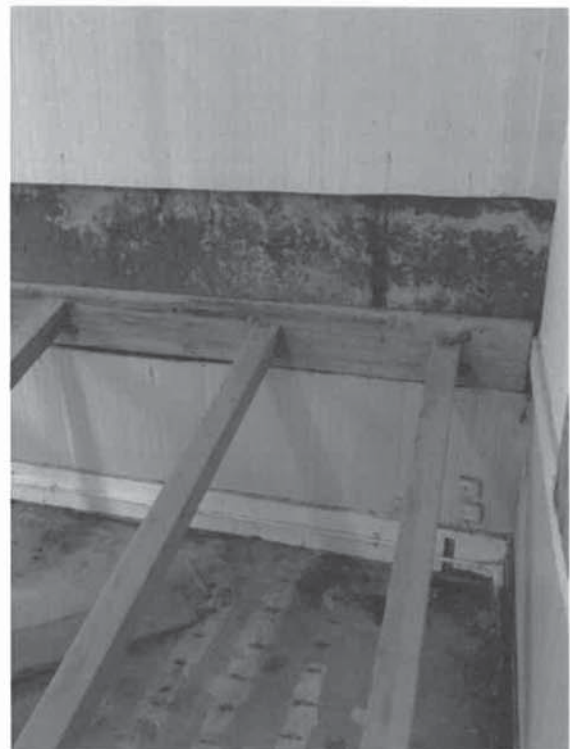
Photo 5 & 6: Close up of the failed retaining wall and insufficient waterproofing which led to the dry rotting floor framing.
