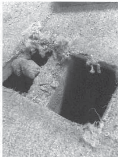
Photo 8/9: This photo shows the damage that wood framing has incurred due to the lack of adequate separation.
