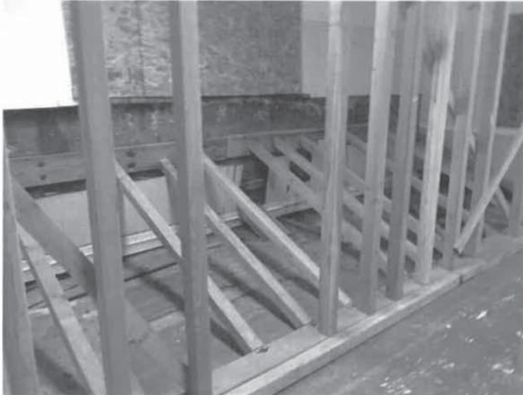
Photo 4: Shoring for the failed retaining wall attached to the existing floor framing.
