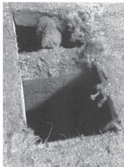
Photo 8/9: This photo shows the damage that wood framing has incurred due to the lack of adequate separation.
