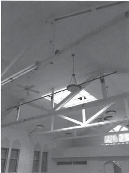
Photo 14/15: These photos show the inadequate truss framing from the interior.
