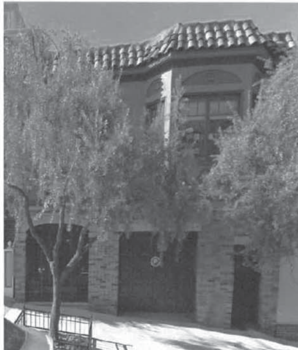
Photo 2: 2-story residential building to the south of the subject property.
